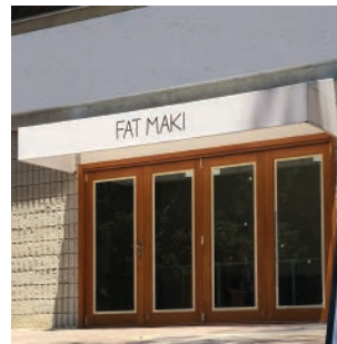
Well Designed and Functional
